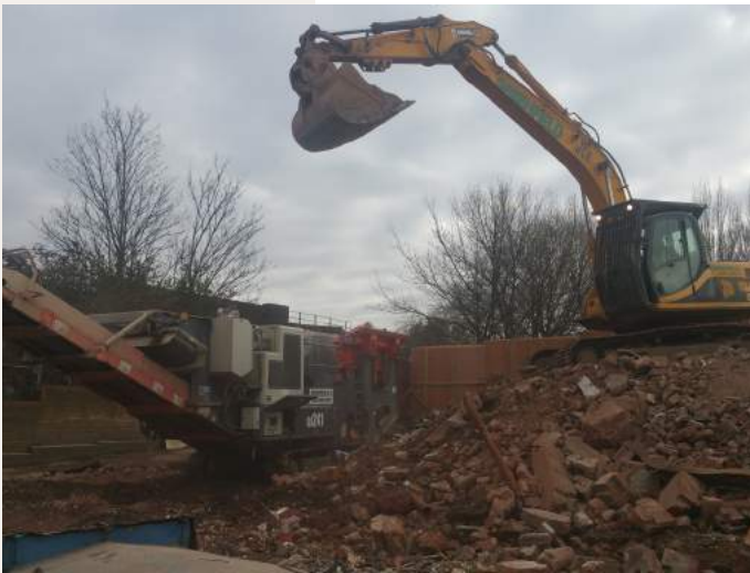
Demolition of Existing Building
