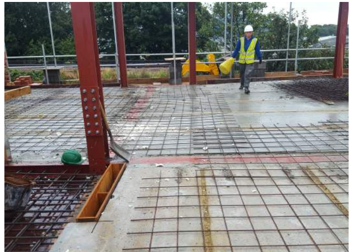
Composite Steel and concrete Structure
