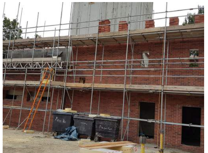
External Brick Work
