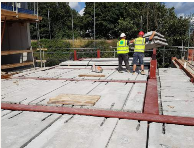
Sub floor- Precast Concrete Planks
