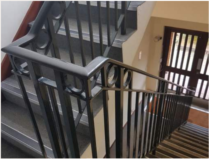
Steel Balustrade to Stairs
