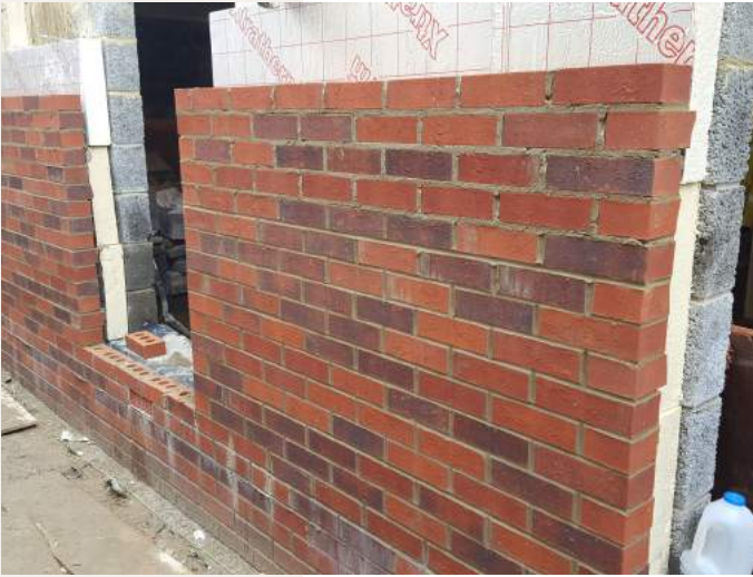
External Cavity Wall
