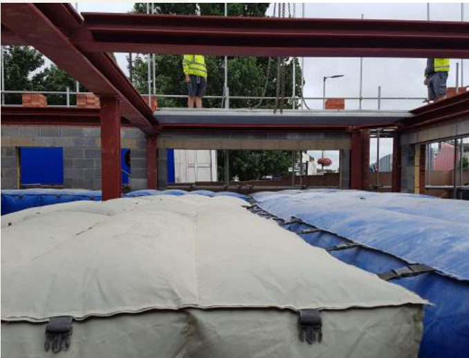
Structural Steel Framework
