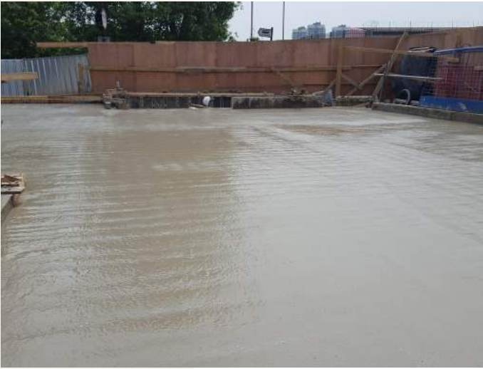
RCC Ground Floor Slab
