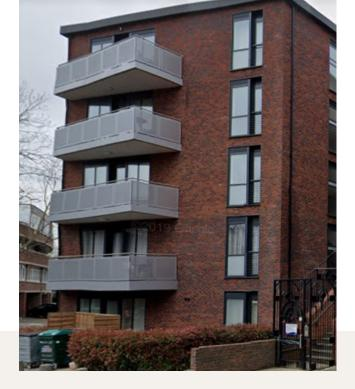
New Build- Construction of 5 storeys mixed (Timber and Steel) frame building following code level4. The development comprised 8 residential apartments. (4x one Bedroom and 4x two bedroom apartments) and 2 commercial offices on the ground floor.
