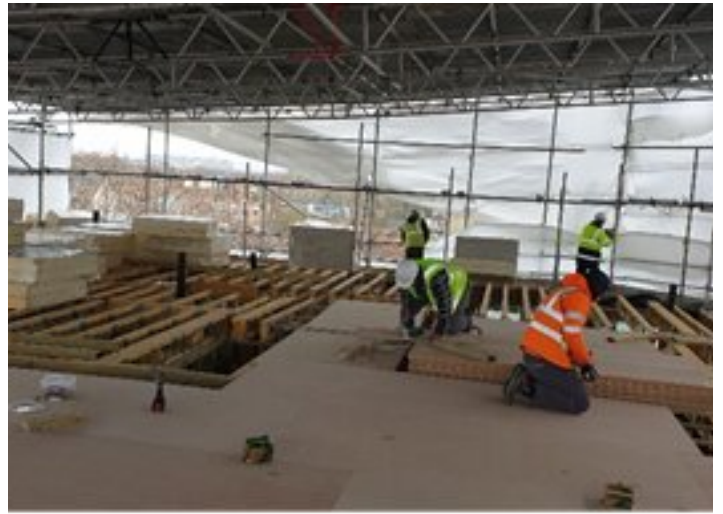
Flat roof Structure- Posi Joists
