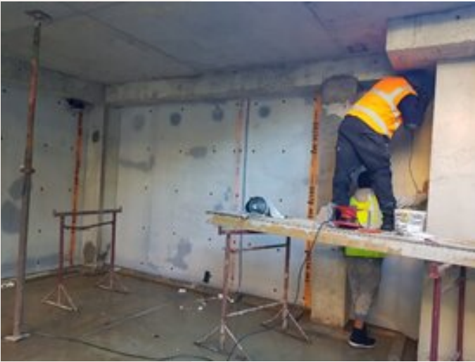
Basement Water Proofing
