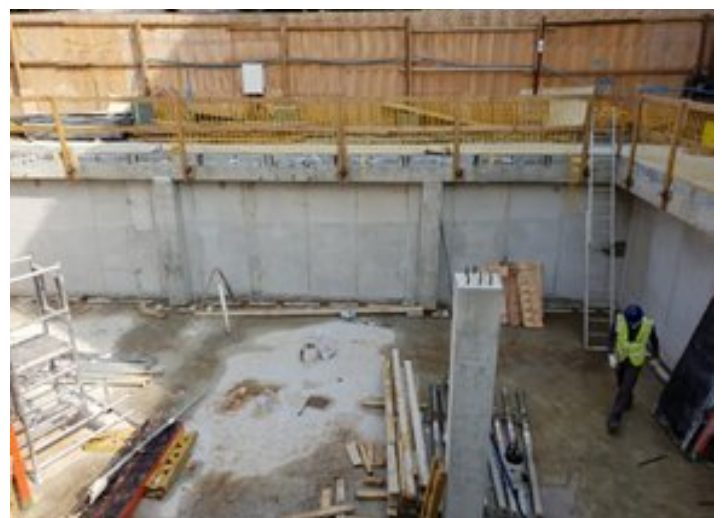
RCC Basement Retaining Walls
