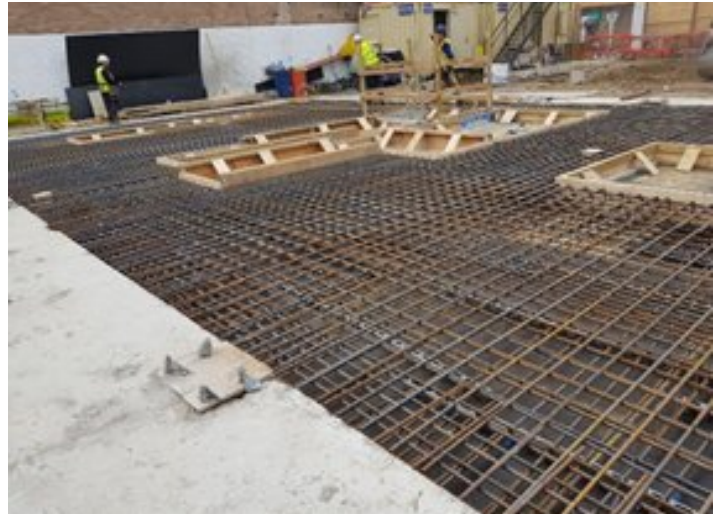
RCC Ground Floor Slab
