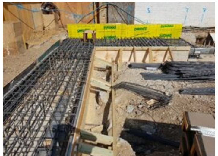
Pile Capping Beam
