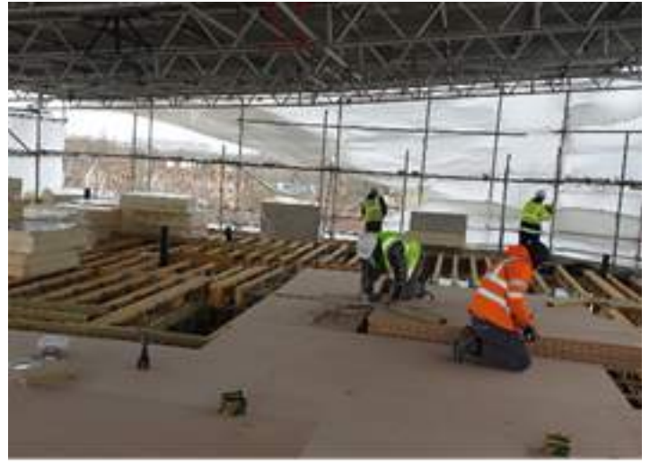
Flat roof Structure- Posi Joists
