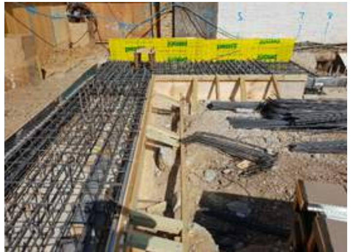
Pile Capping Beam
