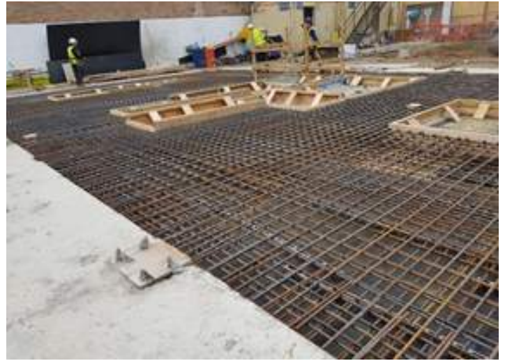
RCC Ground Floor Slab
