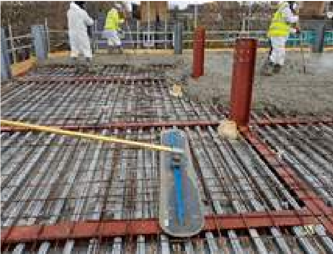
Composite Decking floor
