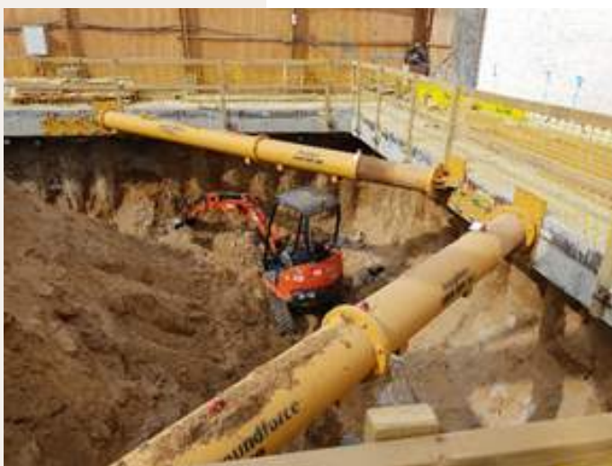
Basement Construction- Temporary Proping
