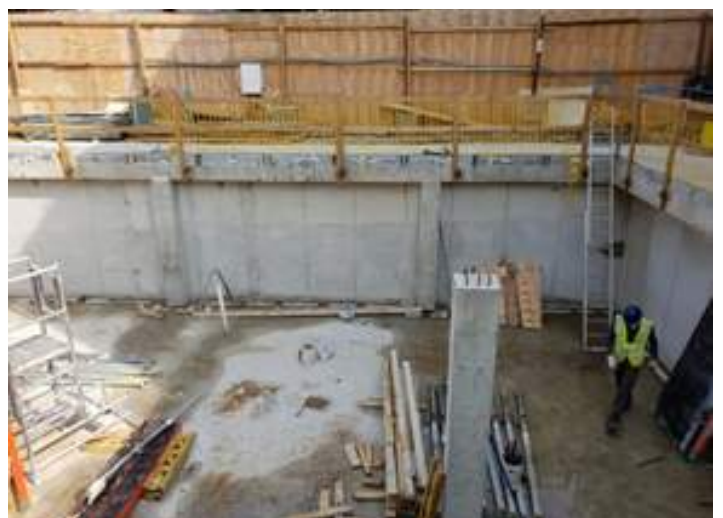
RCC Basement Retaining Walls
