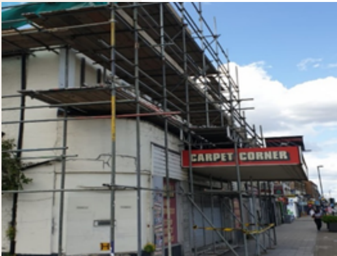
Demolition of Existing Building
