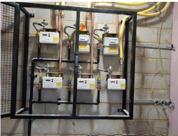
Gas Meter Installed
