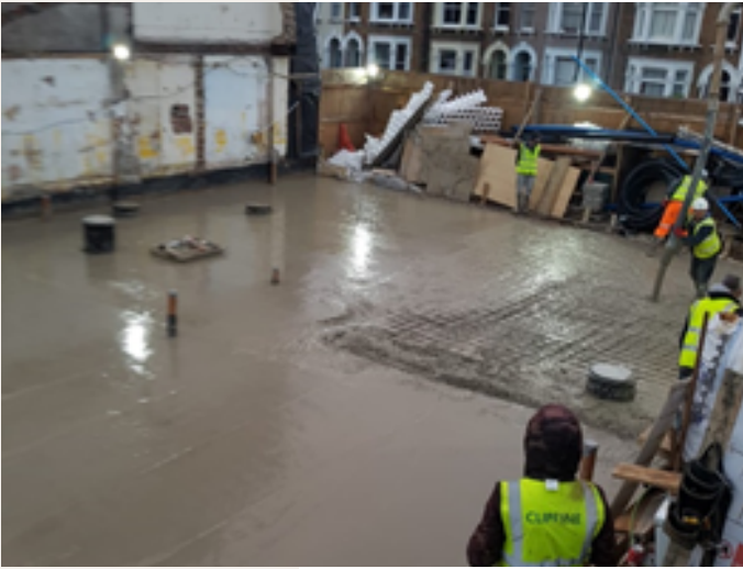
RCC Ground Floor Slab
