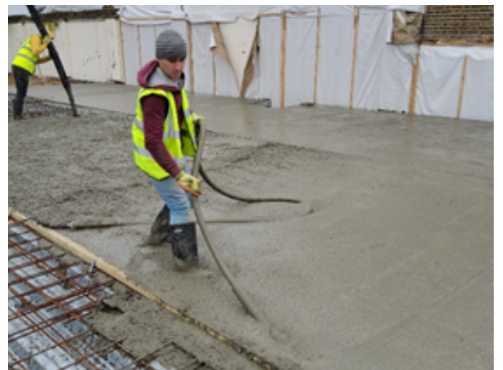
Sub floor- Concrete on Metal Decking
