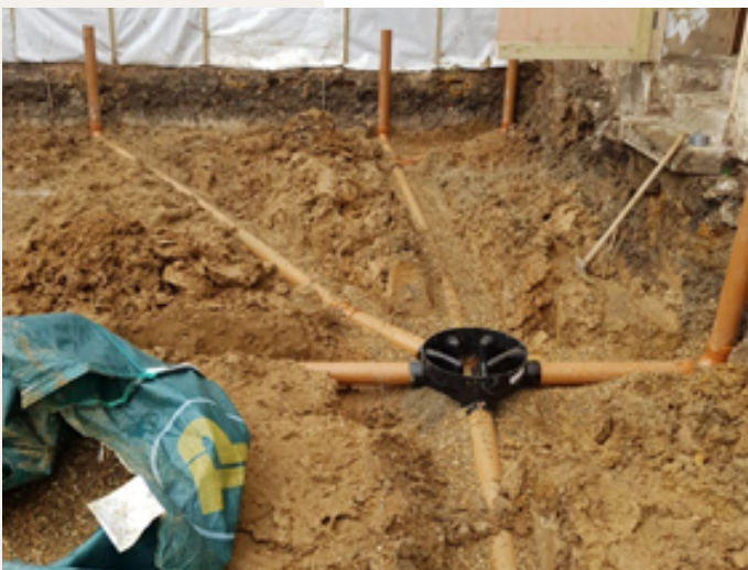
Below ground drainage works
