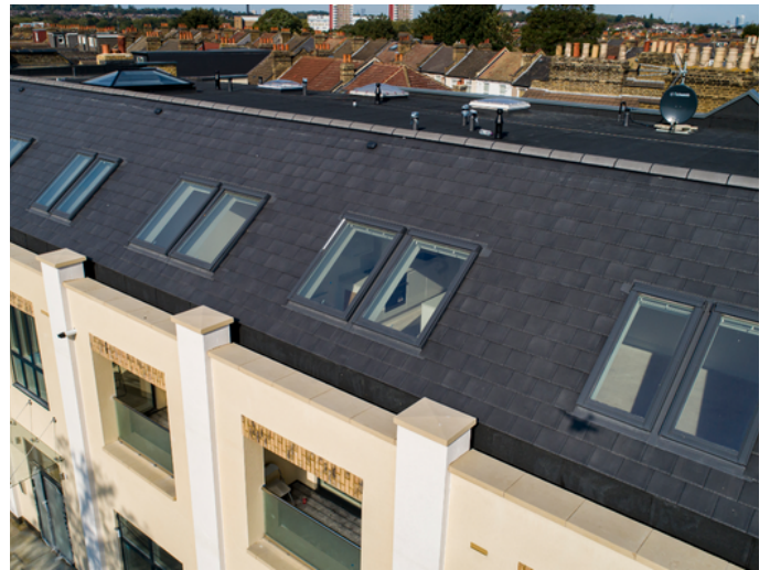
Finished Pitch Roof
