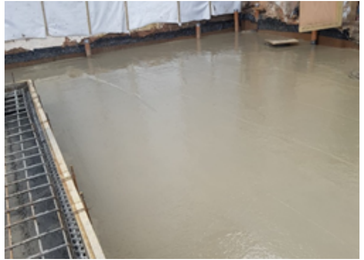
RCC Ground Floor Slab
