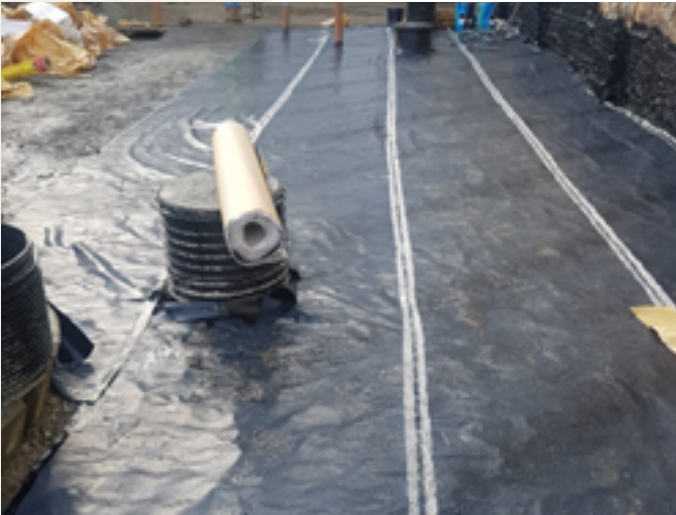
Ground Floor Slab Waterproofing
