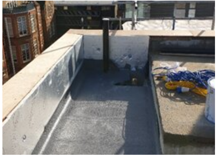
Roof Waterproofing
