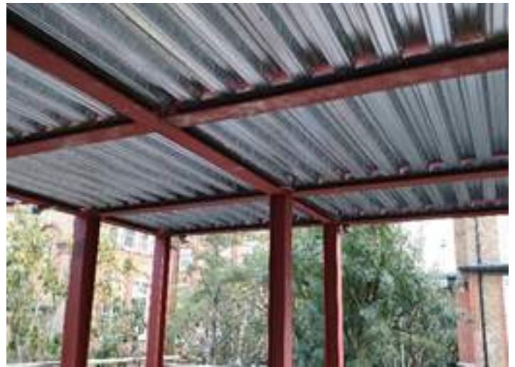
Subfloor-Metal decking
