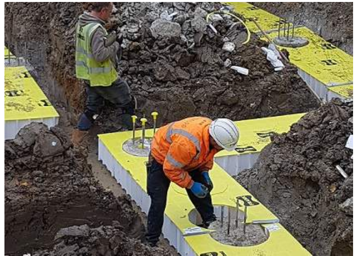
Capping & Ground Beams
