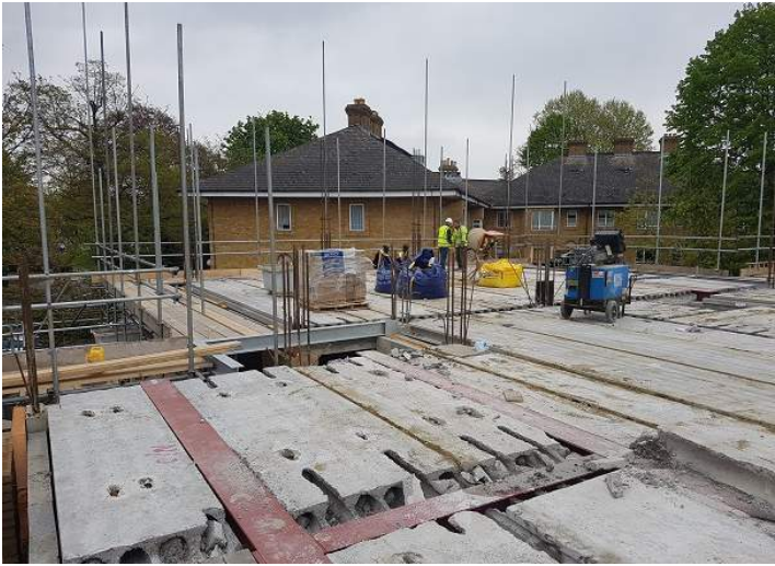
Sub floor-Precast concrete planks
