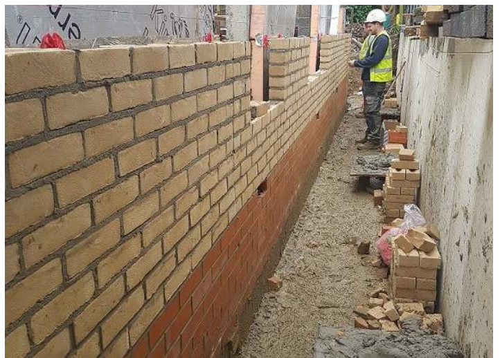
External Cavity Wall-Brick Work
