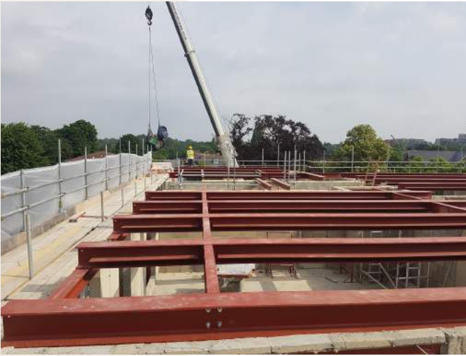
Structural Steel Framework
