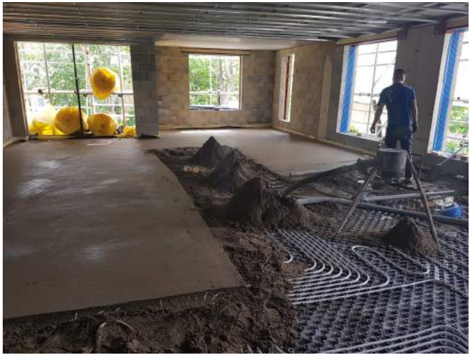
Sub floor- UFH & Screeding
