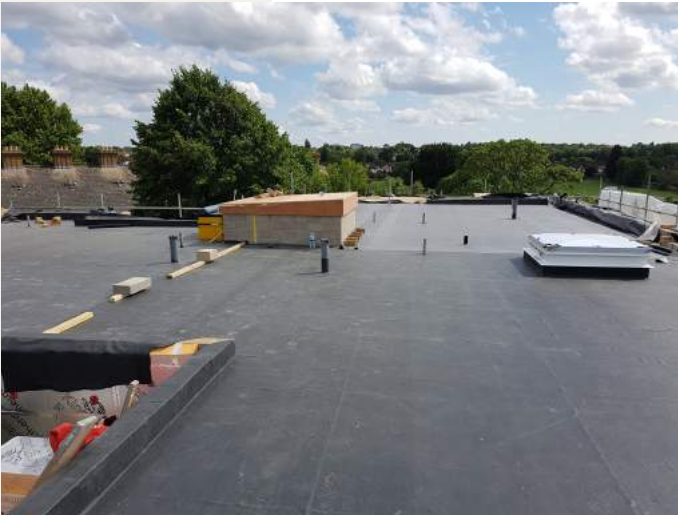
Roof Waterproofing
