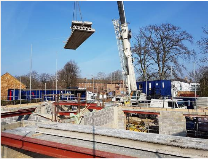
Sub floor- Precast concrete planks
