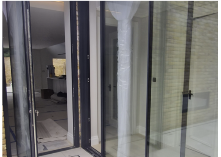
Aluminium Windows Installation
