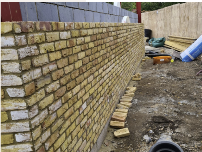
Masonry Work- External Brick Cladding
