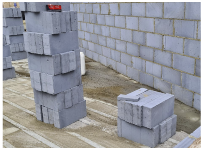
Masonry Work- Internal Block Work
