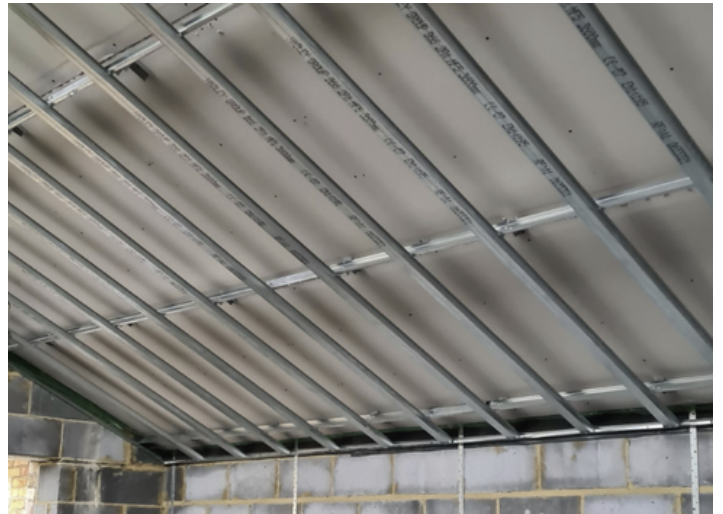
Metal Stud-Ceiling Work
