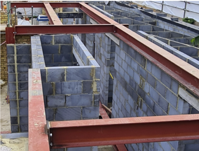
Structural Steel Work
