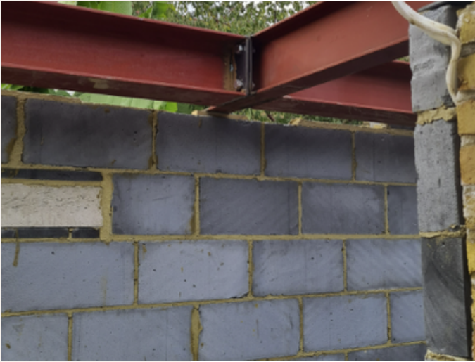
Masonry & Structural Work
