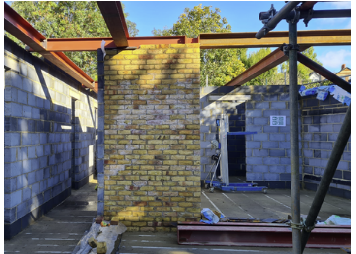
Structural Steel Work
