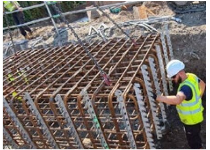
Pile Capping Beam
