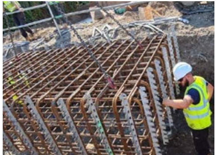
Pile Capping Beam
