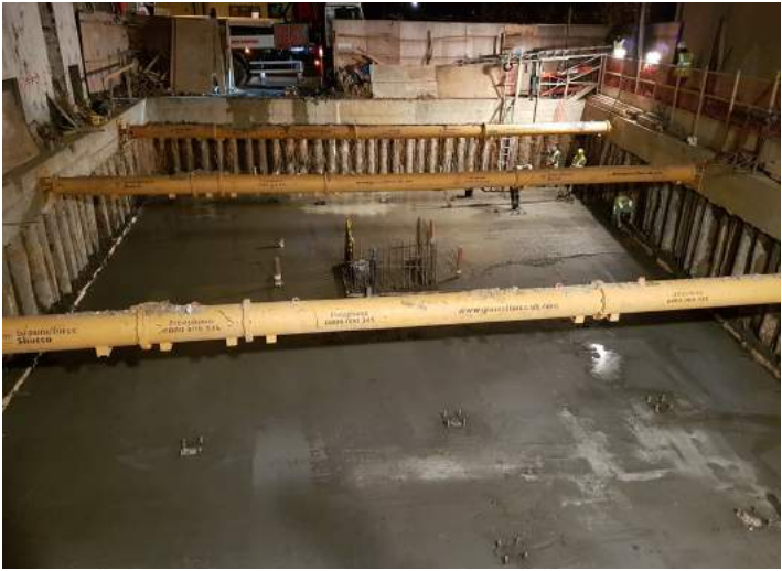
RCC Basement Floor Slab
