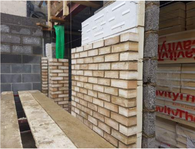
External Cavity Wall
