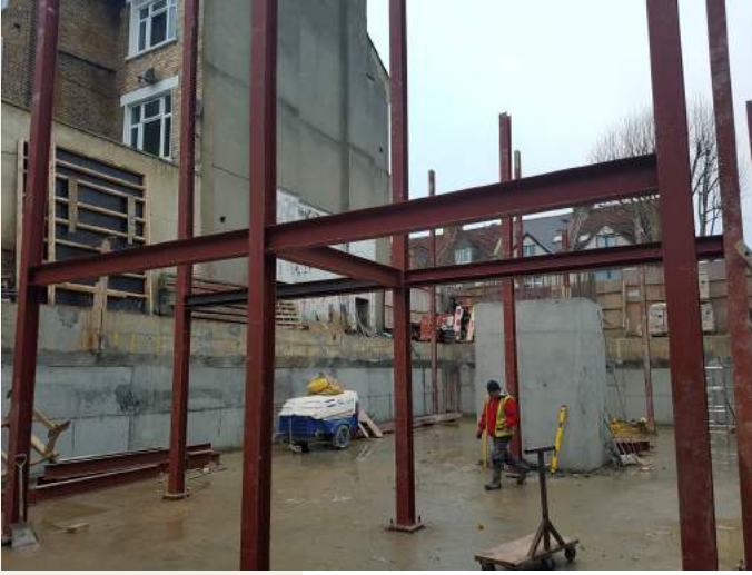
Structural Steel Framework
