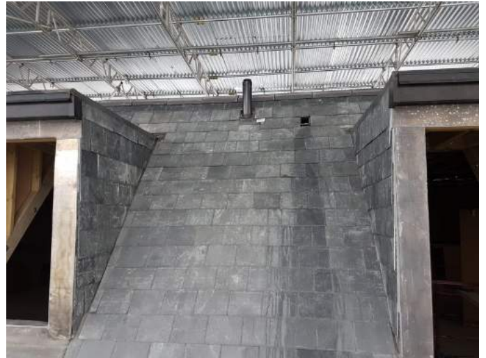
Finished Pitch Roof
