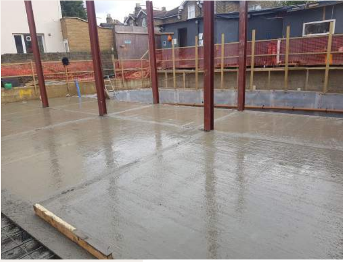
Sub floor- Concrete on Metal Decking
