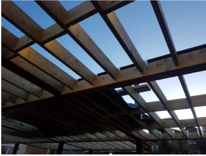
Sub floor- Timber Joists
