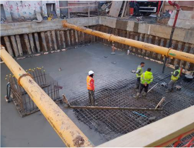
RCC Basement Floor Slab
