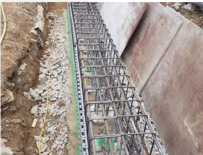
Capping Beam-Basement perimeter
