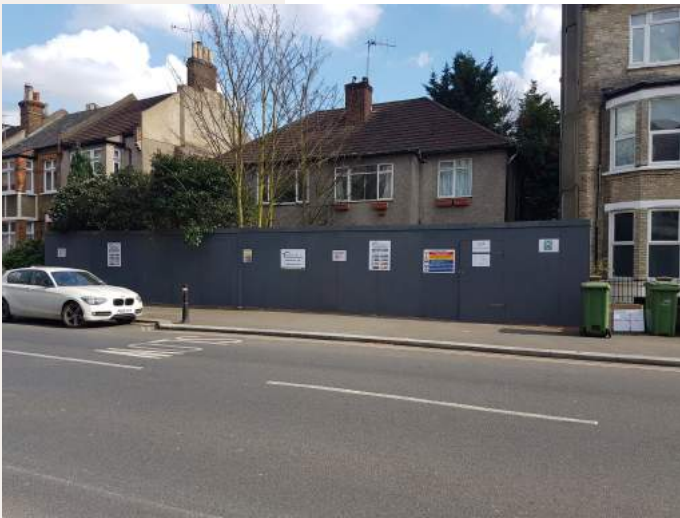
Demolition of Existing Building
