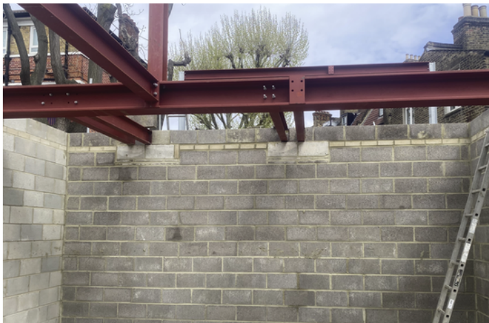
Block & Structural Steel Work Block B
