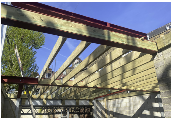
Sub-floor Timber Joists Block B
