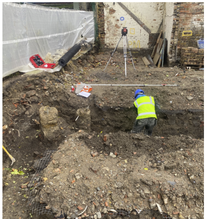
Excavation for Ground Beams
