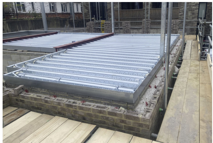
Concrete Metal Decking Flat 1- Block B
