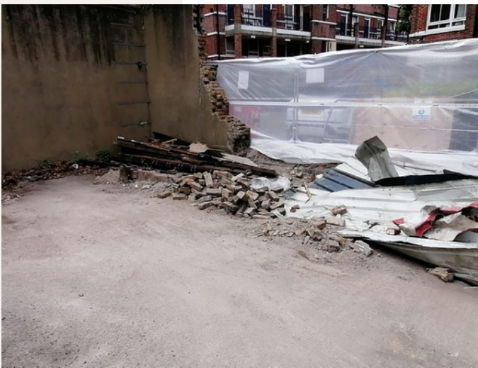
Demolition of rear wall
