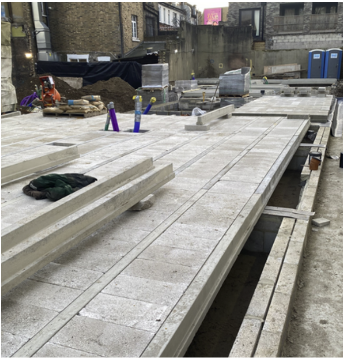
Beam & Block Floor Block B
