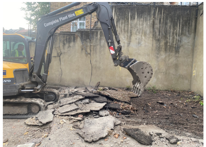
Pile Probing Works
