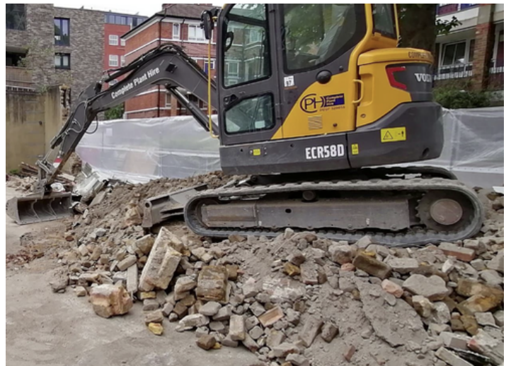
Demolition of rear building
