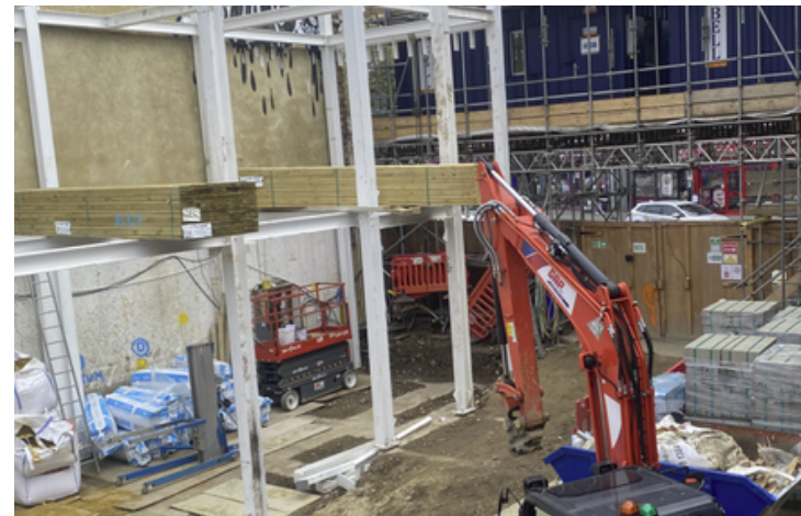
Structural Steel Works Block A
