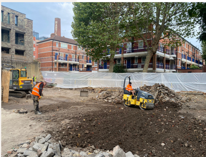
Pile Probing Works
