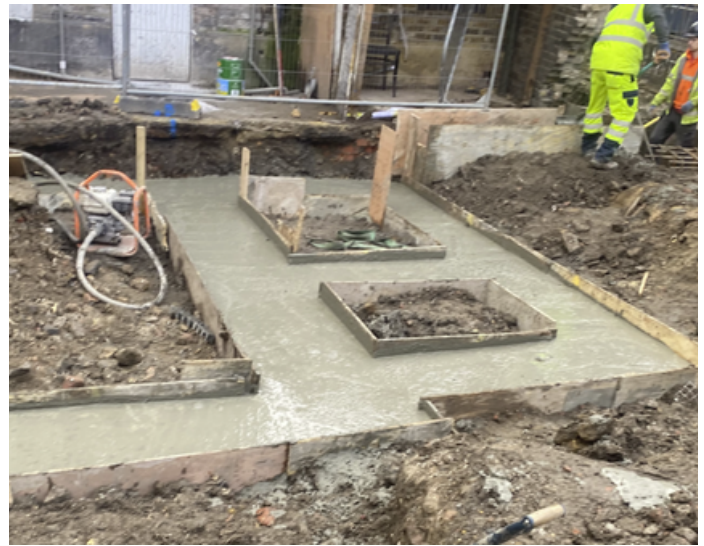
Ground Beams
