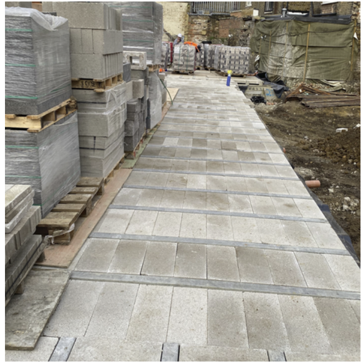
Beam & Block Floor Block B
