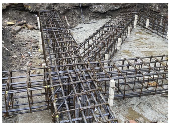
Reinforcement Ground Beams
