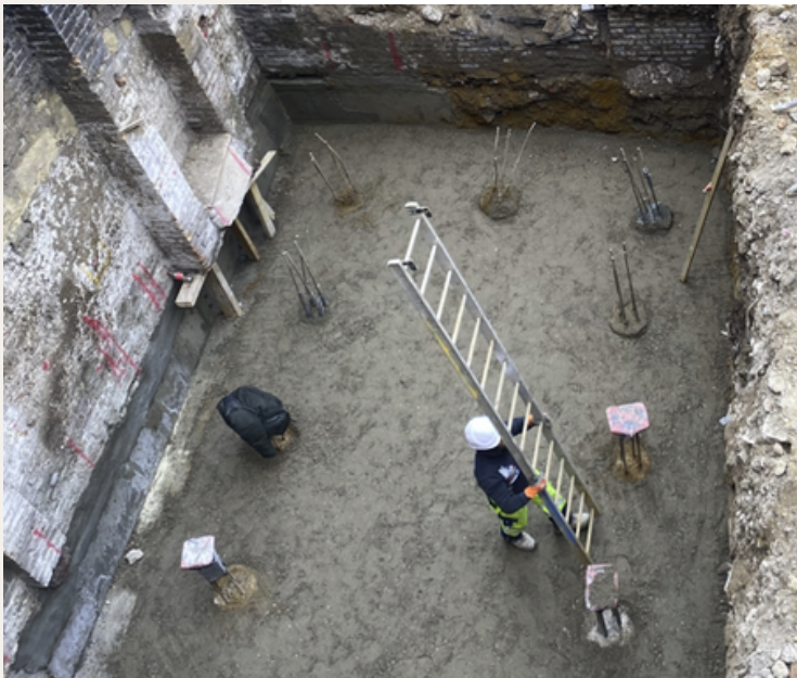
Basement Pile cutting
